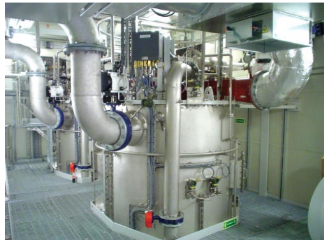
Typical view of the versatile Moss Inert Gas Generator. This example is from an offshore installation.
