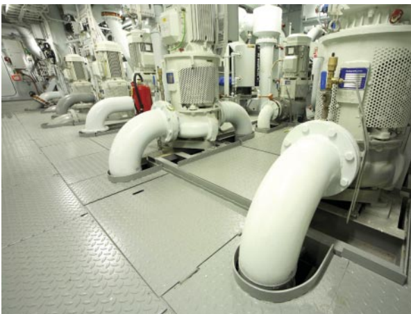
Typical Hamworthy CG pump installation onboard vessel
