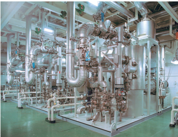
Reliquefaction plant installation onboard 'Sanha' LPG-FPSO
