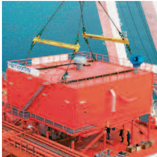
VOC RECOVERY PLANT
