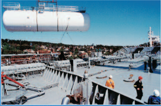
400m 3 VOC fuel tank being installed onboard Shuttle tanker 'Navion Viking'
