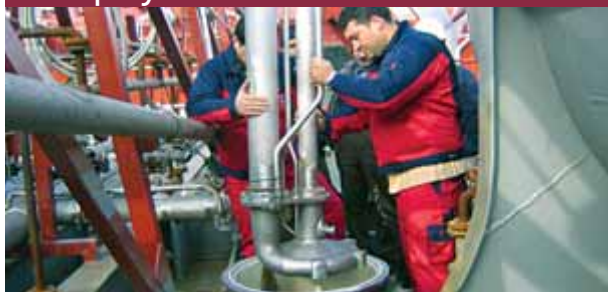
Deepwell cargo pump being installed in Turkter Shipyard, Turkey.
