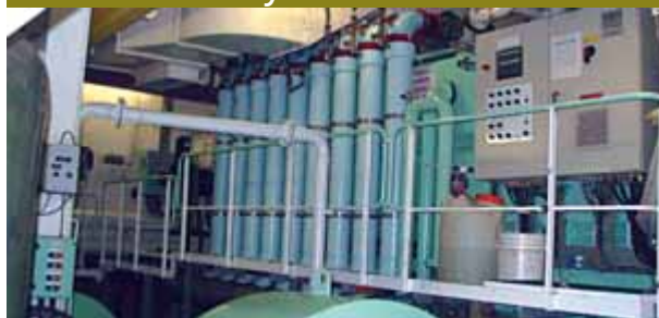
Membrane bioreactor on board Princess Cruises's Dawn Princess.
